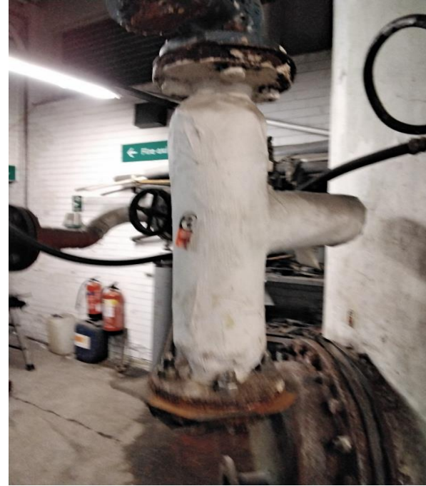
Lagged Pipework
