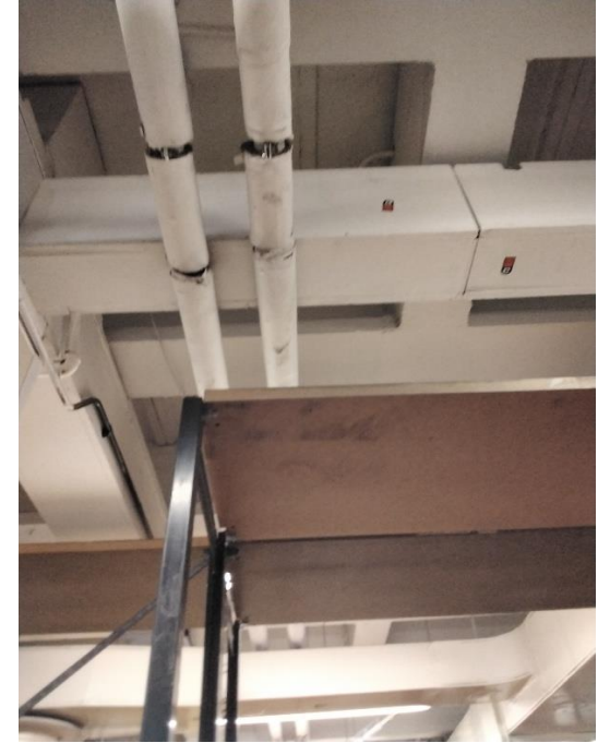
AIB to beams
